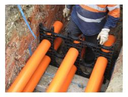
Multiple layers of varying conduit size can be combined in an easy clip construction. No special tools required.
